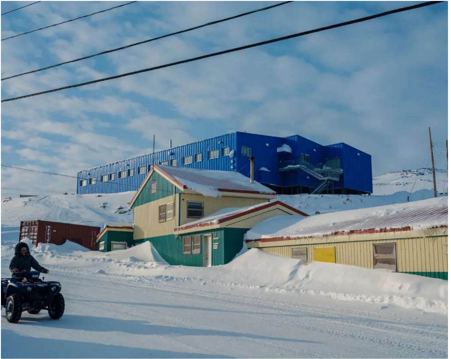
The old Kinngait Studios sit below the new Kenojuak Cultural Center and Print Shop, a $10.8 million facility that opened in 2018. Brendan George Ko for The New York Times
